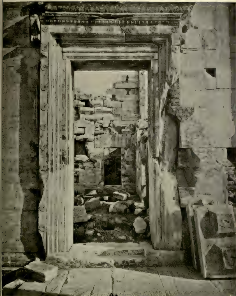
DOOR OF NORTH PORCH (before restoration) Erechtheum, Athens
